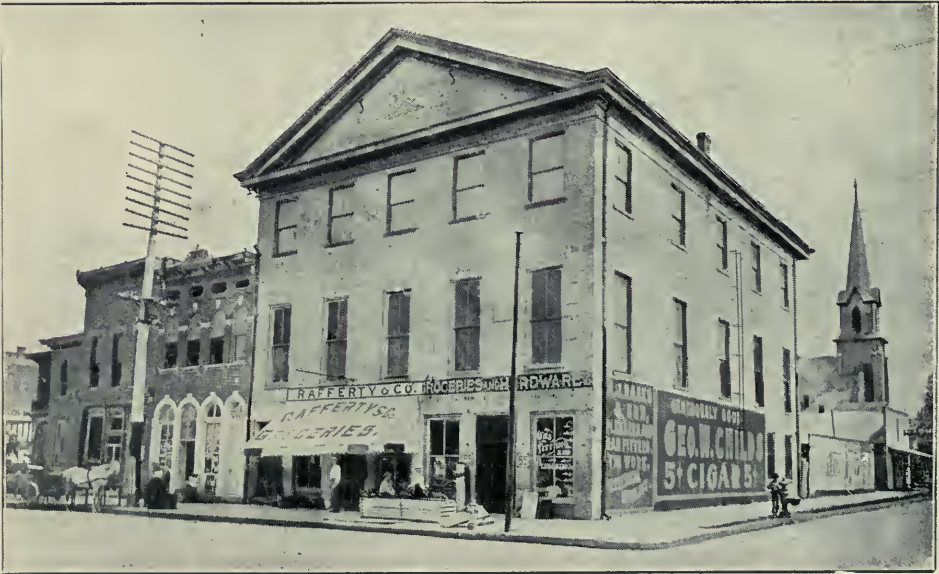
OLD MASONIC HALL, GREENFIELD
