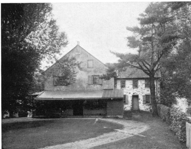
THE ORTHODOX MEETING HOUSE AND SCHOOL BUILDING IN THE REAR
