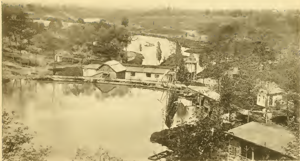
Looking West from Auditorium.
