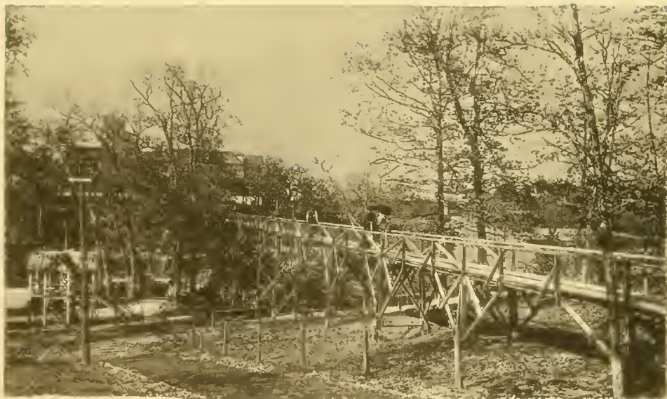
Bridge from Auditorium to Hotel
