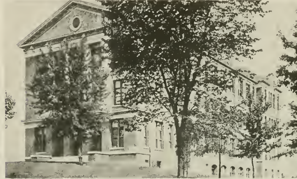
McIVER MEMORIAL BUILDING, BUILT IN 1908
