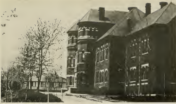
EARLY VIEW OF THE ADMINISTRATION BUILDING
