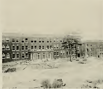
QUADRANGLE UNDER CONSTRUCTION, 1921-23
