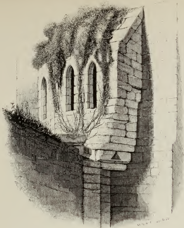
ORIEL OF THE CHAPEL OVER THE GATEWAY, PRUDHOE CASTLE, NORTHUMBERLAND
