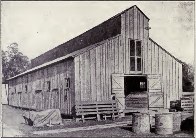
Monitor type winter farrowing house on farm of F. W. Clew, near New Orleans, La.
