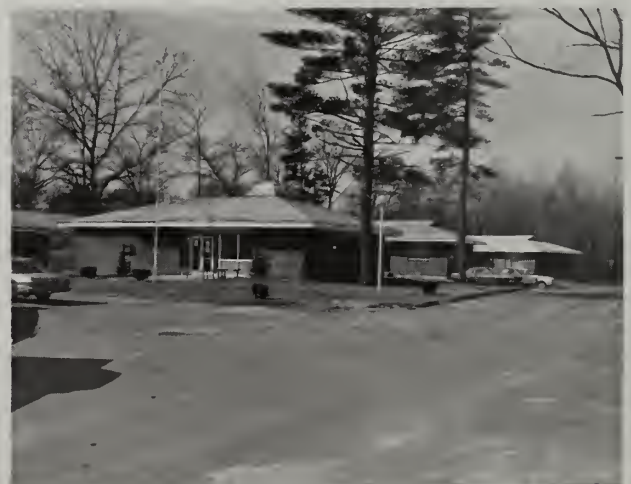
Community Building Elderly Housing
