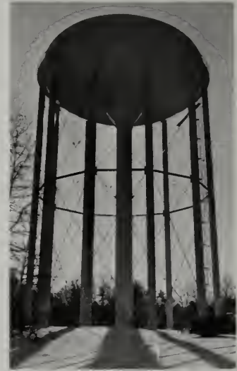
1,000,000 gallon water Storage Tank
