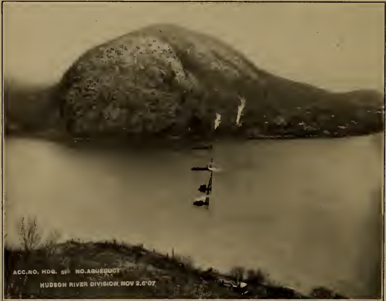
FIG. 1. View of the Storm King Crossing, looking southwest from Breakneck Mountain, while the drilling was in progress from the scows. The east shaft is just below the hill in the near foreground.
