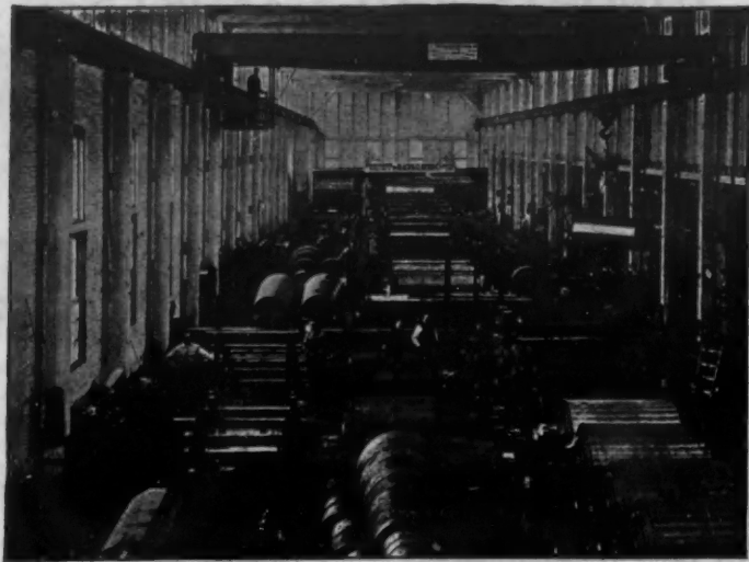
Erecting Department of the Black & Clawson Co. Shops, 50 ft. x 270 ft.
