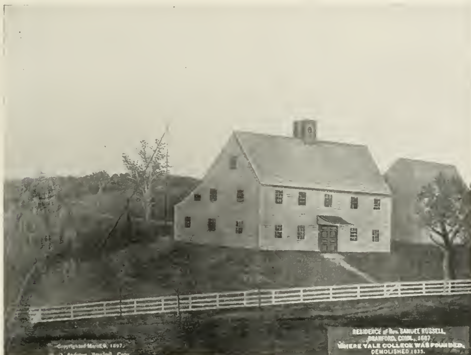
OLD HOUSE IN BRANFORD
