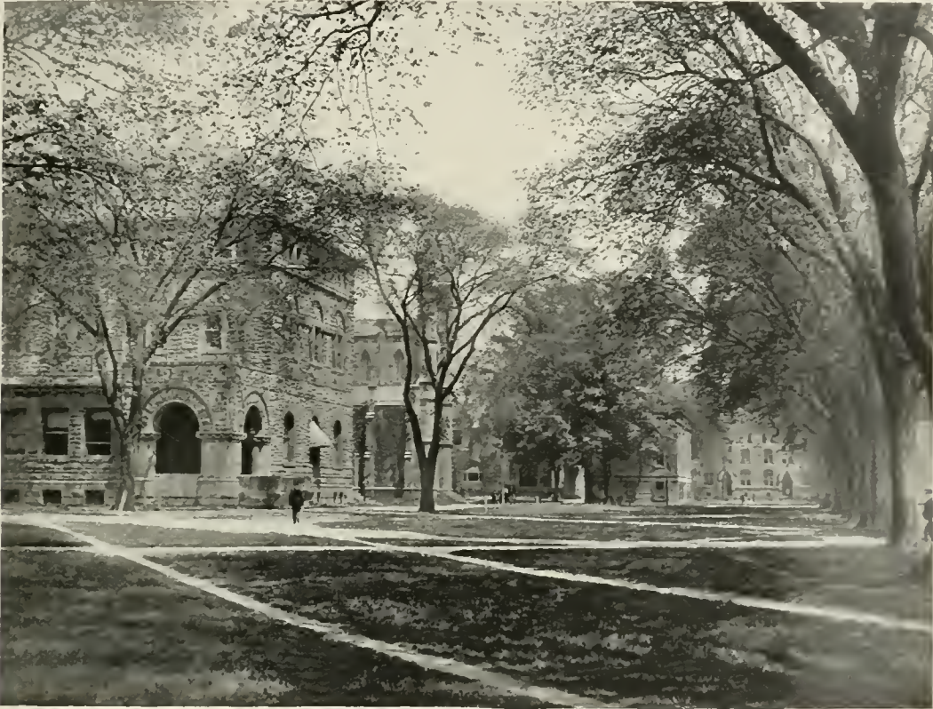
REAR VIEW OF CAMPUS, LOOKING SOUTH
