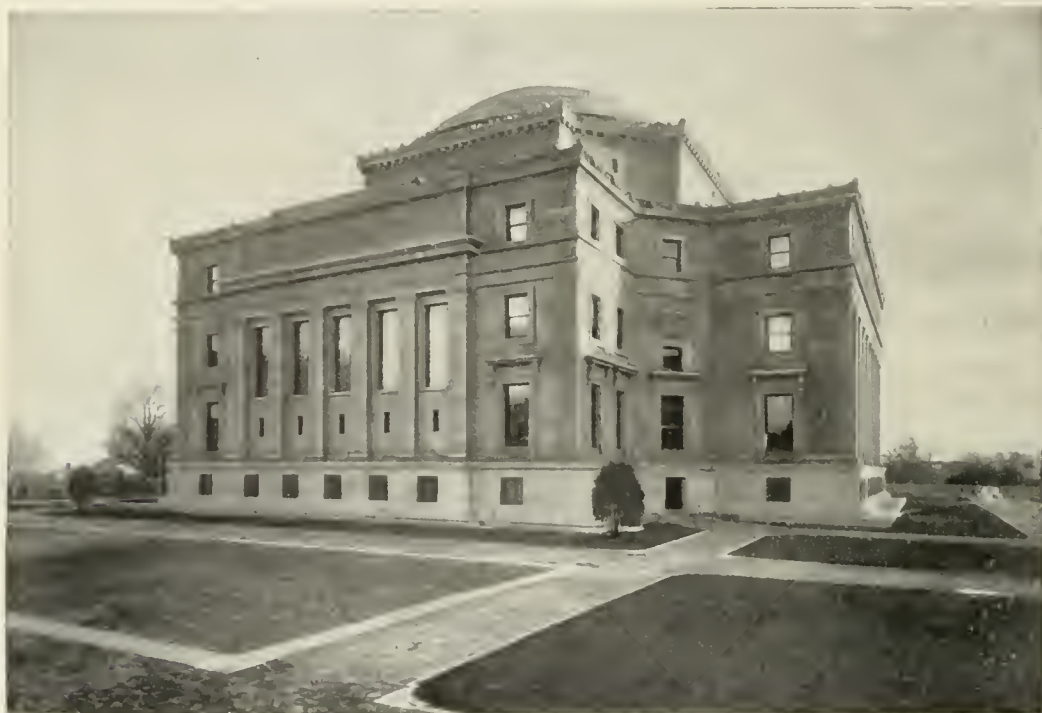
LAW SCHOOL WING OF LIBRARY BUILDING
