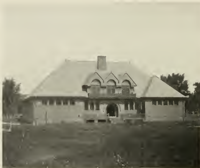
CAREY BUILDING, HOLMES FIELD
