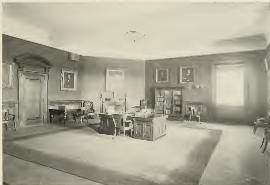
PRESIDENT'S ROOM, LIBRARY BUILDING
