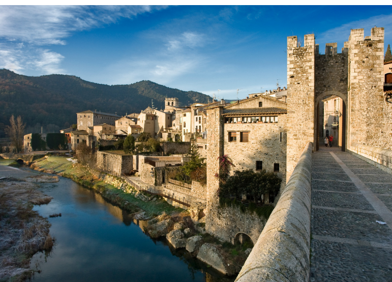
Photographer: Mikipons Monument: Medieval fortified village of Besalú Location: Besalú, Spain
