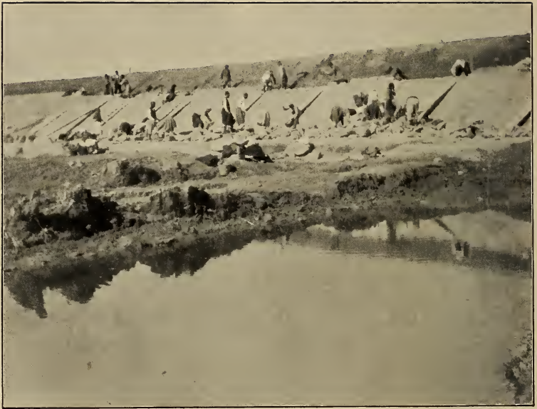
WALL OF NEW RESERVOIR, ACHERITOU
