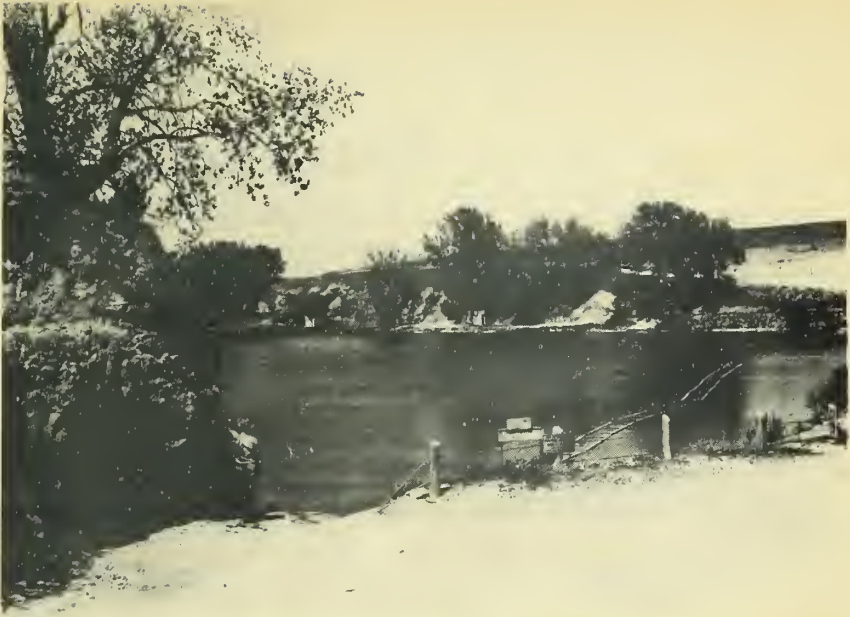
Figure 3.--Bluff of loess at the south end of Wellfleet dam.
