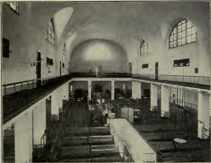
MAIN WAITING ROOM, IMMIGRATION BUILDING, NEW YORK CITY.
