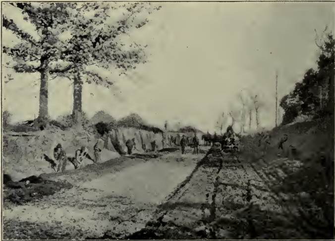
PREPARING THE ROADBED.
