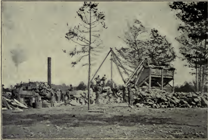
PREPARING THE MATERIAL.
