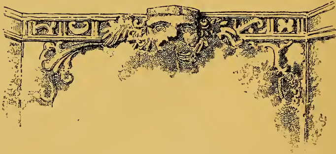
DECORATION OVER DOOR-WAY.
