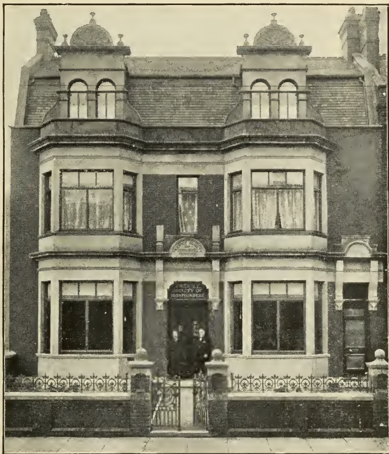
PRESENT GENERAL OFFICE.
