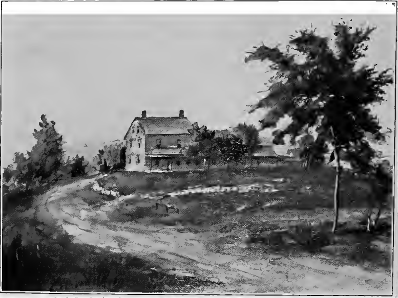
THE JOSIAH BENNETT HOUSE, MAPLE STREET.
