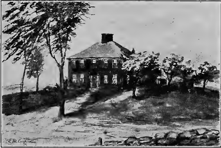
ITHAMAR BRIGHAM HOMESTEAD.
