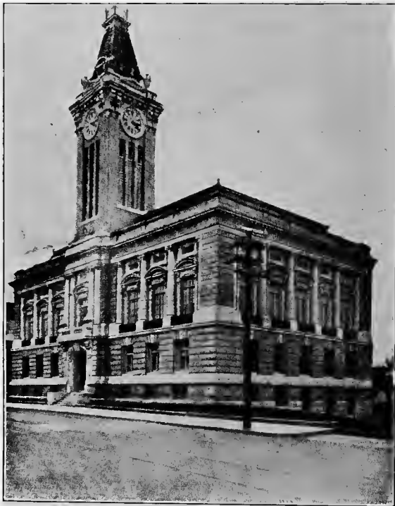
MARLBOROUGH CITY HALL.
