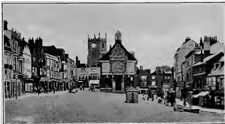
HIGH STREET AND TOWN HALL, OLD MARLBOROUGH, ENGLAND.
