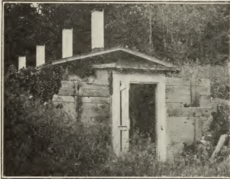
FIG. 7.—This cellar belongs to Ira Bartlett of East Jordan, Mich. He had some heavy losses in the cellar, which he attributed to bad stores and old bees. When asked if he didn't have too much ventilation, as shown by the ventilators, he admitted that that might be true. The sides and embankments are not covered by a roof, as will be noticed, and the result is that the temperature varies.
