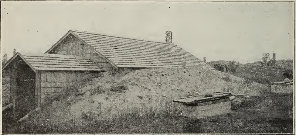
FIG. 4.—This belongs to L. C. Gordon of Bellaire, Mich., and apparently has the same defect as Fig. 3. The owner said that in this 12 x 20-foot bee-cellar last winter he wintered 151 colonies, without the loss of a colony. According to David Running's idea the roof should have extended over the side embankment. But these embankments are made up of sand that dries out very quickly; and, in spite of the fact that it is not covered, it makes a good insulator. This cellar has the ventilation recommended by Mr. Running.
