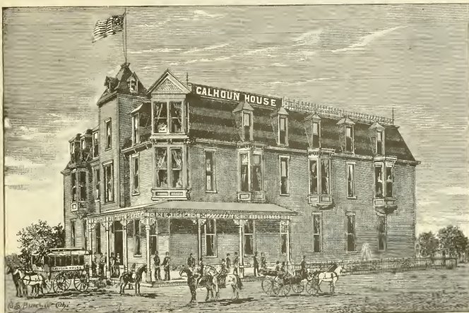
THE NEW CALHOUN HOUSE, NESS CITY.
