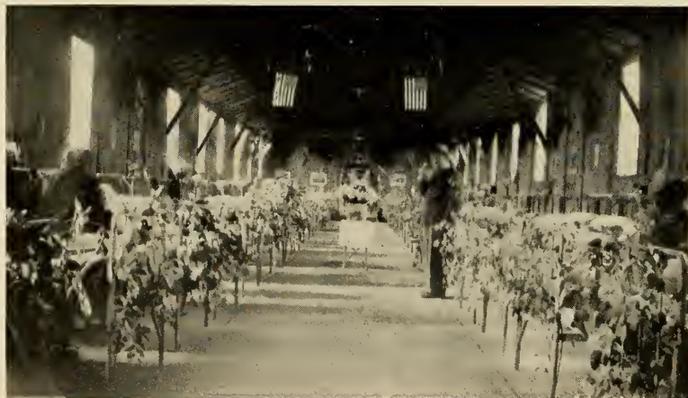
INTERIOR OF A WARD
