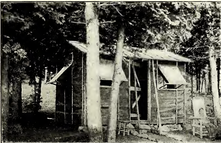
THE COMPLETED HOUSE, VERY COMFORTABLE AND QUITE WEATHERPROOF
