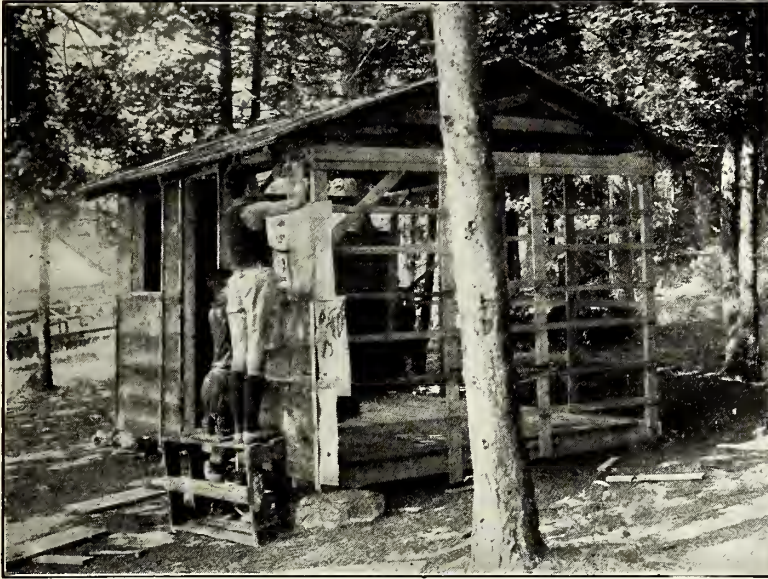
PUTTING ON THE PAPER, WITH GLUE AND LATHS, AND PAINTING IT GREEN
