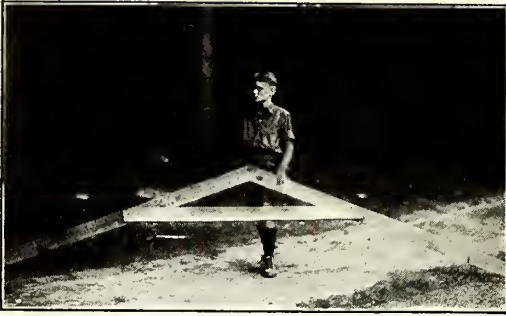
ONE OF THE THREE "A" PIECES THAT SUPPORT THE ROOF. NOTE THE NOTCHES THAT ENGAGE THE FRONT AND BACK WALLS
