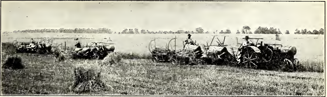
BINDERS, EQUIPPED WITH GRAIN SHOCKERS AND PULLED BY 10-20 HORSEPOWER TRACTORS
