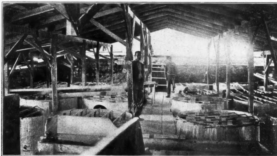
CRYSTALLIZING TANKS, BORAX WORKS, HARNEY COUNTY, OREGON.
