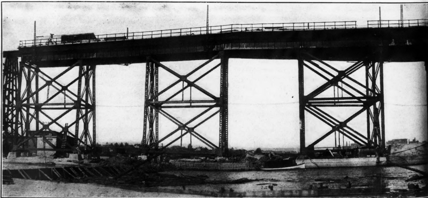
NEW NORTHERN PACIFIC ORE DOCK, AT SUPERIOR, WIS. S. S. SAUNDERS TAKING THE Dock is of steel and concrete, 684 ft. long; steel approach, 300 ft. long; timber approach, 4200 ft. long; steel used in dock, 35,700 tons; bins have circular fronts, are equipped
