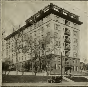
GARAGE IN CONNECTION
