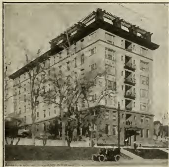
GARAGE IN CONNECTION
