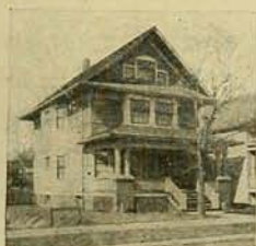
A No. A-241 IDEAL Boiler and 461 ft. of 38-inch AMERICAN Radiators costing the owner $215, were used to Hot-Water heat this cottage.
