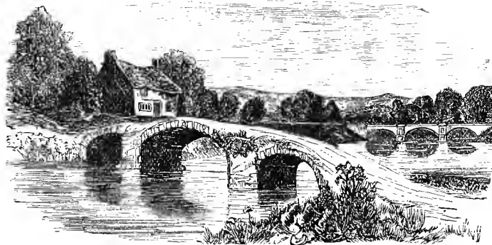
THE HODDER BRIDGE.
