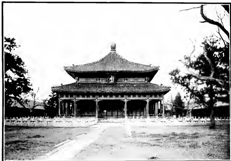
THE IMPERIAL LECTURE ROOM, OLD UNIVERSITY BUILDING
