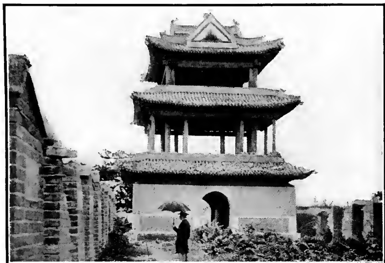
THE WATCH TOWER IN EXAMINATION GROUNDS
