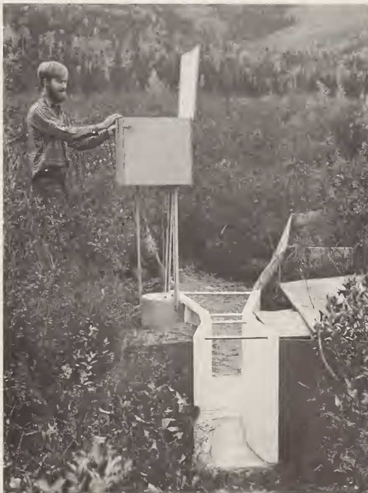
Figure 1.—Parshall flume in C-2 channel; view is upstream. Water-level recorder is in box above the stilling well.
