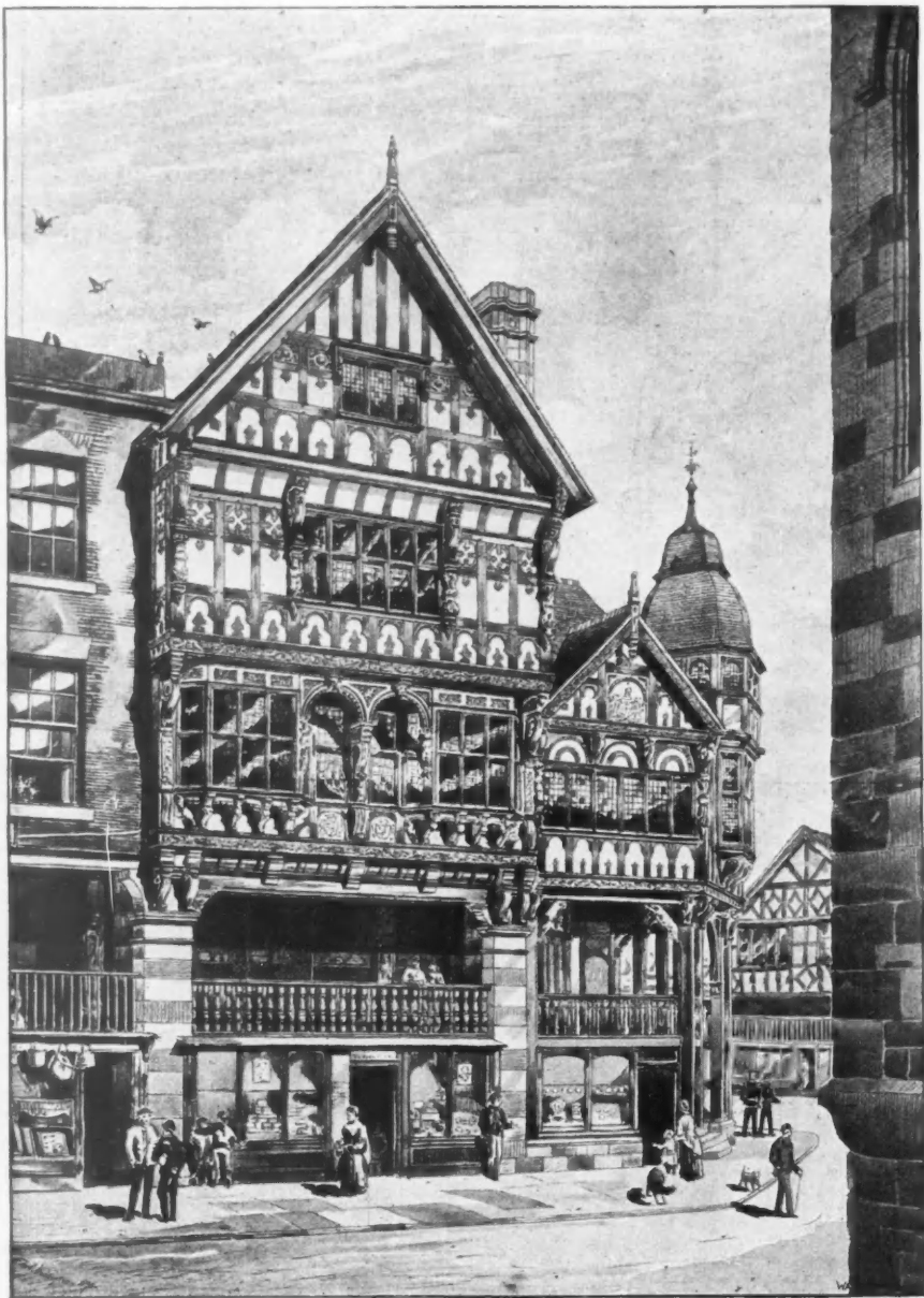
1865. New Buildings at the Cross, Chester, for His Grace the Duke of Westminster, THOMAS M. LOCKWOOD, F.R.I.B.A., Architect.
