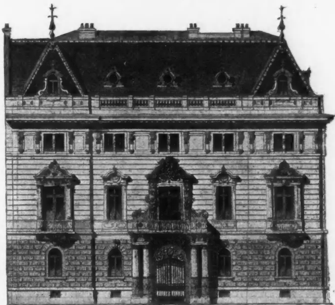
Palace of Baron Albert Wodianer, Budapest, A. v. WIELEMANS, Architect, Vienna.
