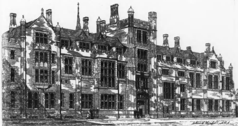
1889. The Church House, View of Front in Dean's Yard , SIR ARTHUR W. BLOMFIELD, A.R.A., Architect.
