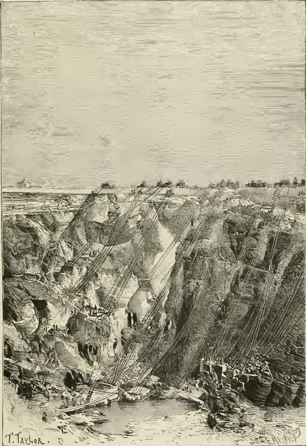
Fig. 47. KIMBERLEY: APPEARANCE OF THE MINE IN 1880.
