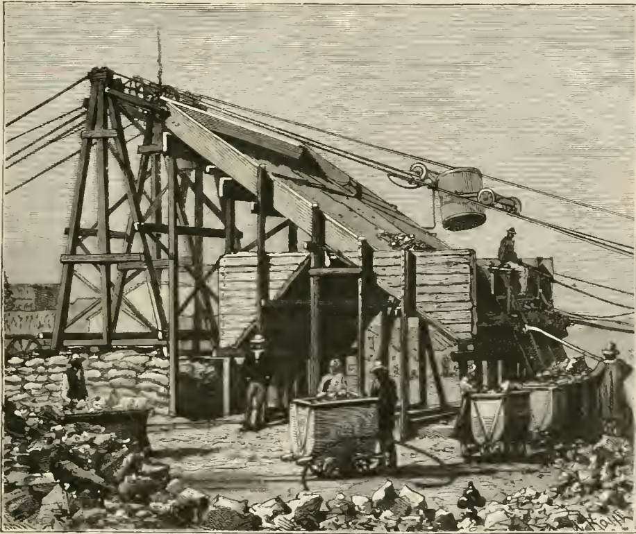
Fig. 48.—APPARATUS FOR RAISING THE DIAMANTIFEROUS EARTH.
