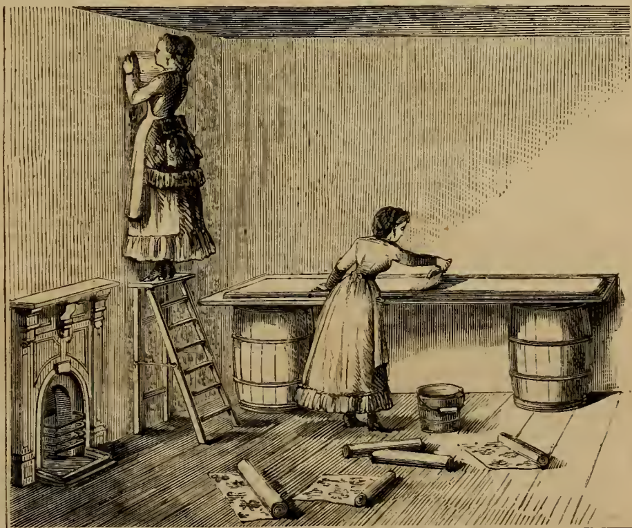
Fig. 3.—PASTING AND PUTTING ON WALL-PAPER.
