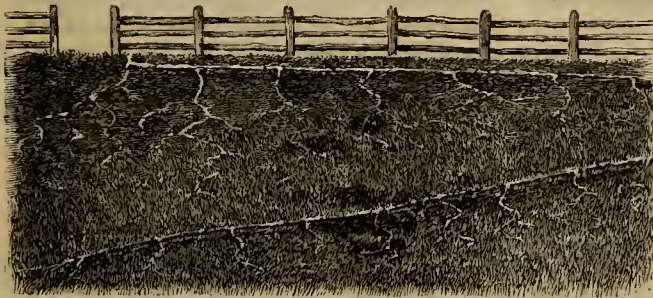
Fig. 2.—IRRIGATING A HILL-SIDE.
