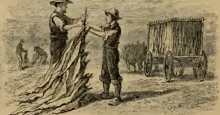
Fig. 4.—STRINGING AND LOADING.
