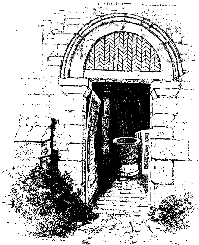
DOORWAY, SOUTH SIDE OF LINLEY CHAPEL.
