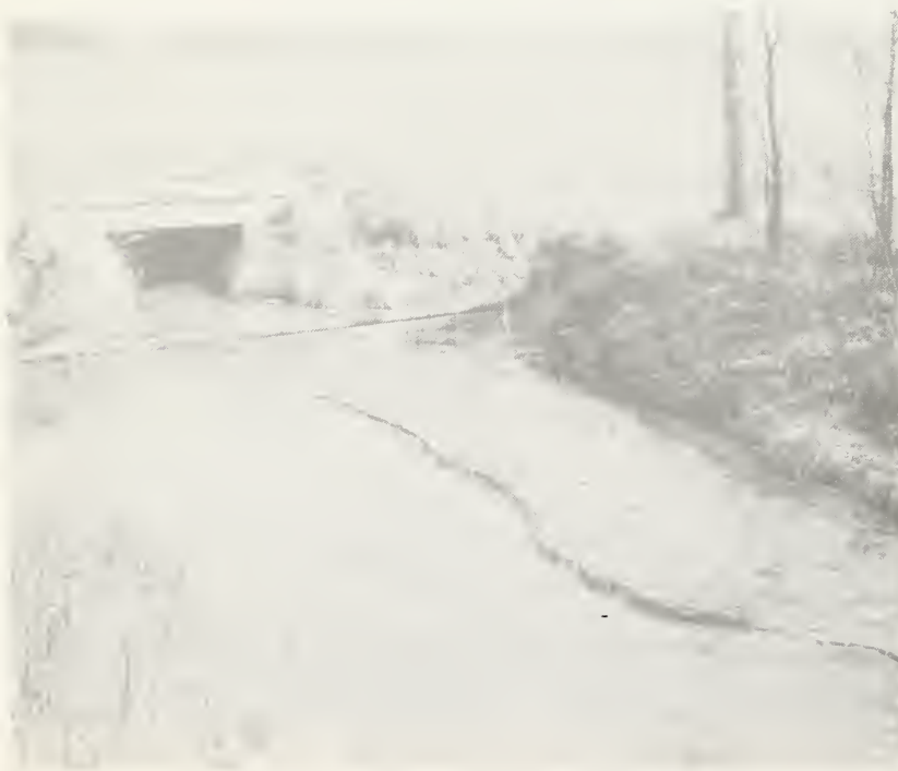
Sediment restricts flow and causes downstream damage. See Exhibit 3.
