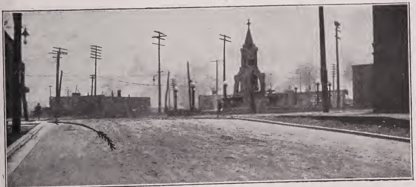
Turn LEFT, 92d Street, South Chicago. Follow trolley to bridge. Next photo six-tenths of a mile.
