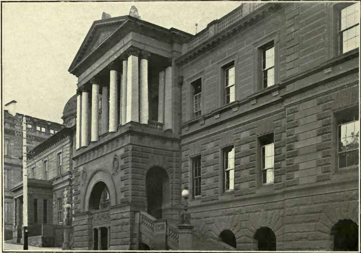
GABO GRANITE COLUMNS AND SYDNEY SANDSTONE. (THE TREASURY BUILDING, SYDNEY, NEW SOUTH WALES.)
