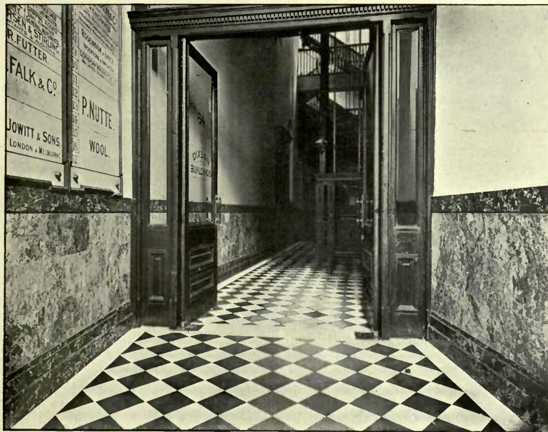
CALEULA MARBLE DADO. (DIXSON BUILDINGS, SYDNEY.)
