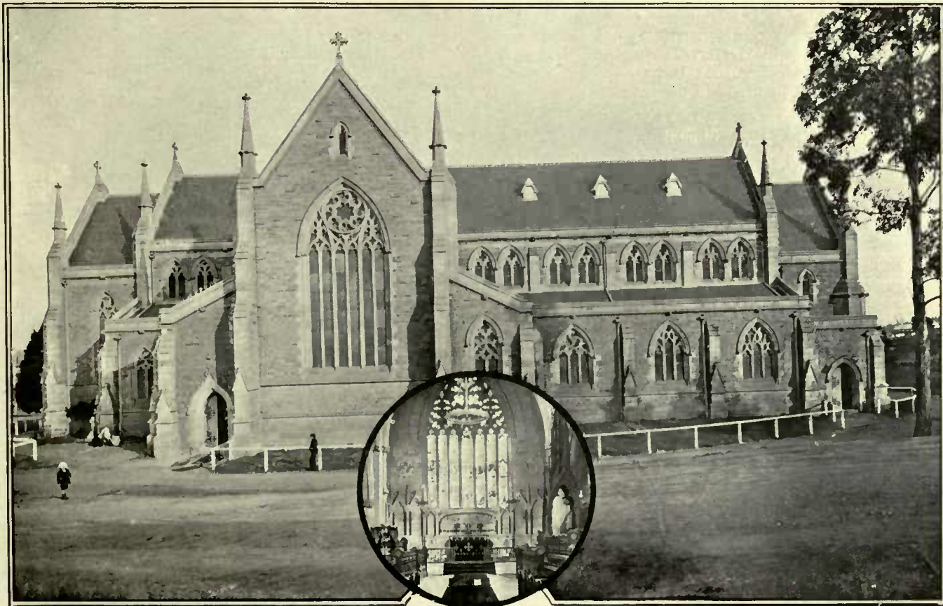
MARULAN SANDSTONE. (ST. SAVIOUR'S ANGLICAN CATHEDRAL, GOULBURN.)
