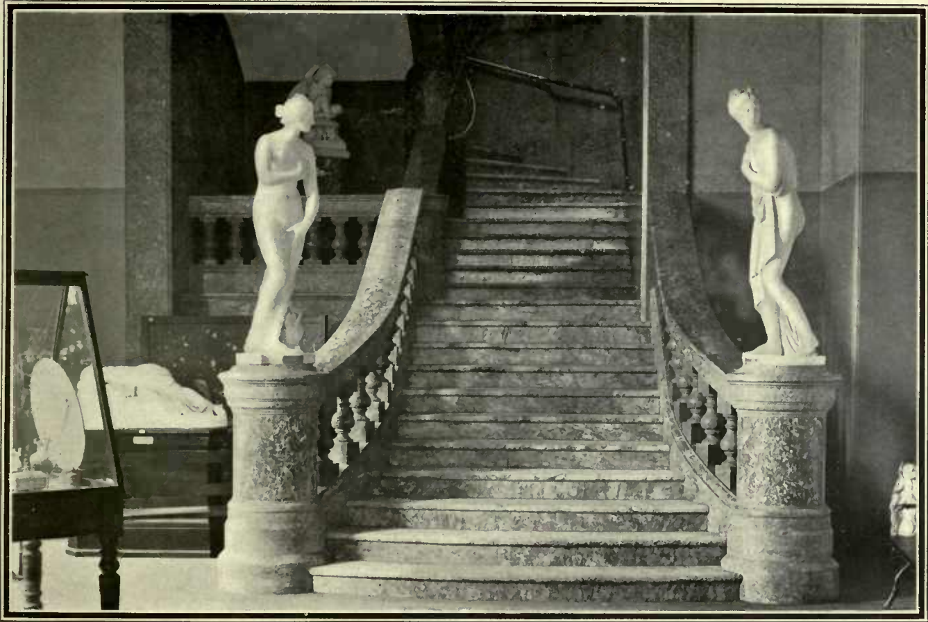
NEWEL SHAFTS OF ROCKLEY MARBLE. RAIL OF FERNBROOK MARBLE. STEPS OF BORENORE MARBLE. BALUSTERS, MOLONG MARBLE. (STAIRS, NATIONAL ART GALLERY, SYDNEY.)
