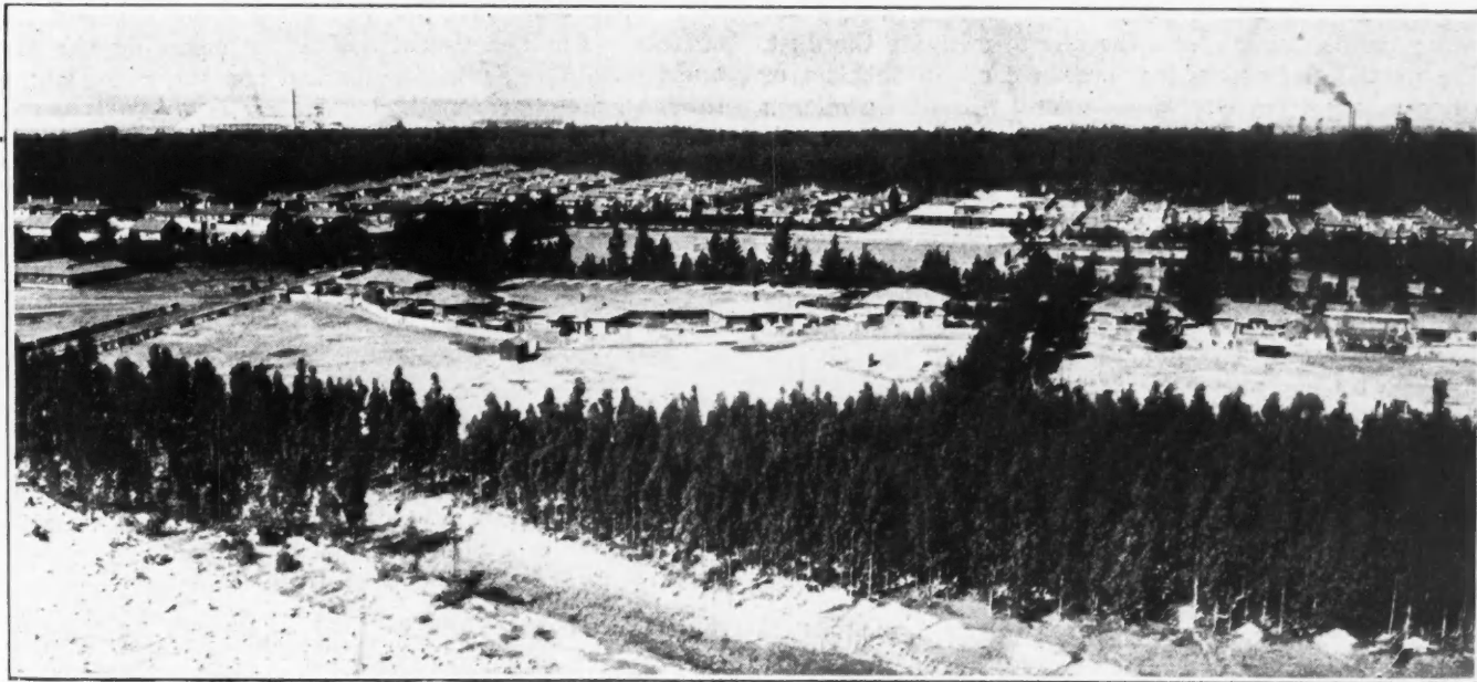
General view looking south from New Modderfontein, No. 12 shaft
