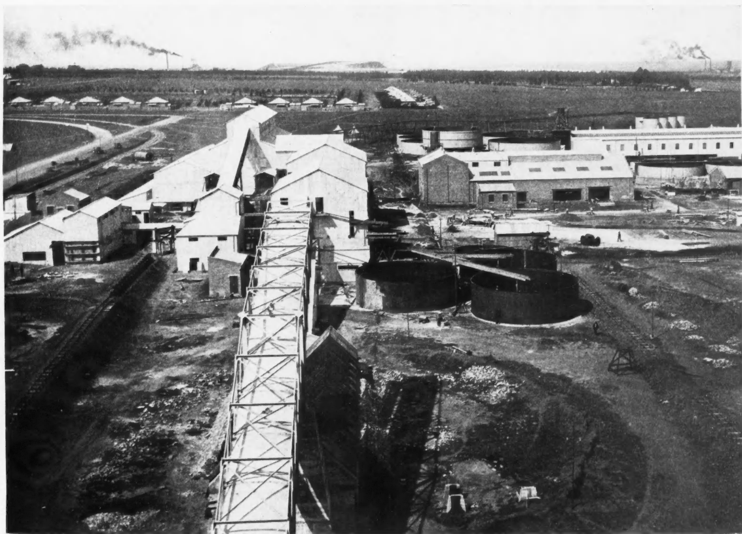
The West Springs Mill on the Rand Stamp milling and amalgamation have been superseded in this new plant
