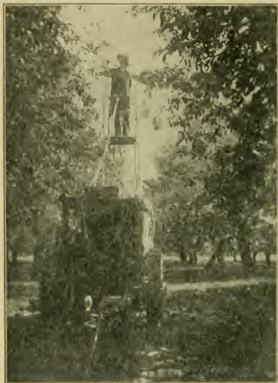
A POWER SPRAYER ADAPTED TO LARGE TREES. A gasoline engine gives uniformly high pressure.
