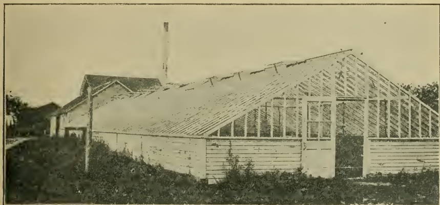
A GREENHOUSE SUITABLE FOR FORCING PLANTS.
