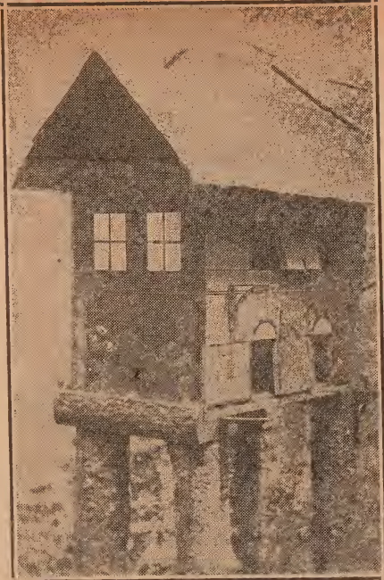
Pigeon Loft built by Moller—The iron braces and huge posts are massive for such a tiny structure.
