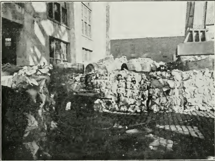
Sorted refuse baled ready for shipment.
