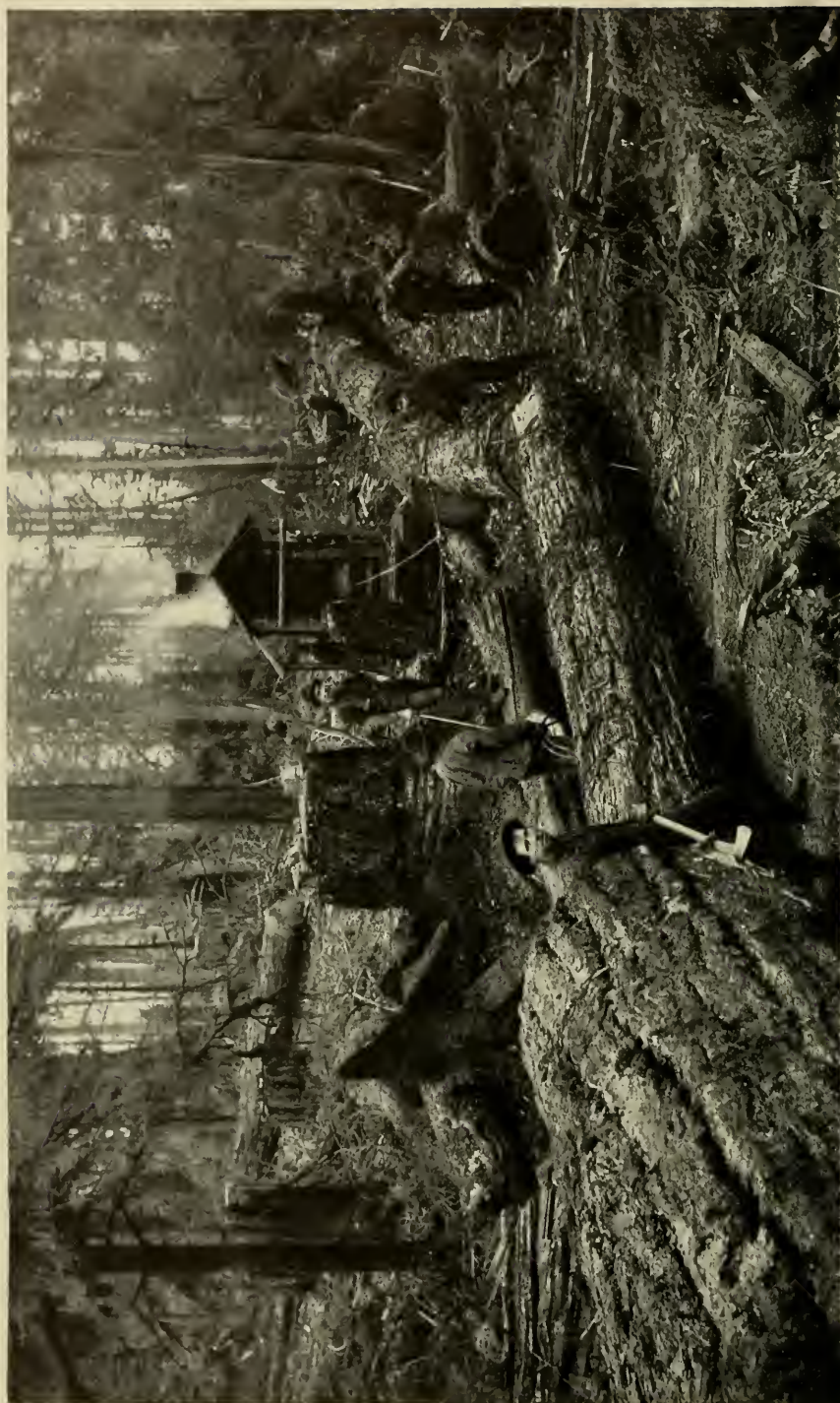
The remarkable donkey-engine yanking the big timber through the woods
