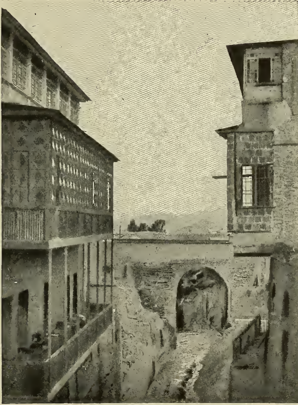
Buildings overlooking a stream that runs through La Paz.
