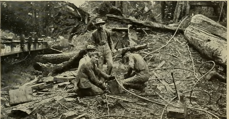
The "riggers" crew repairing cables.
