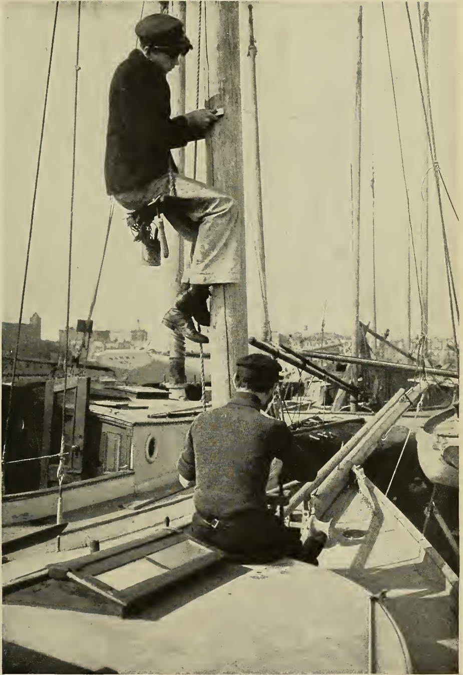
Scraping the mast, preparatory to a fresh coat of varnish.
