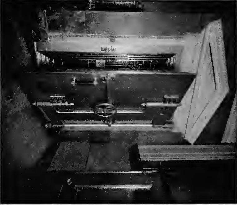
OUTSIDE VIEW OF VAULT.
