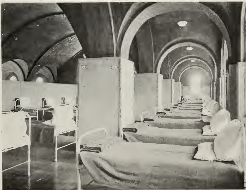
Gallery of Grant Hall, showing the added second floor and the method of protecting the walls and pillars.
