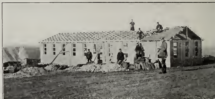
CONSTRUCTING A LABORATORY HUT
