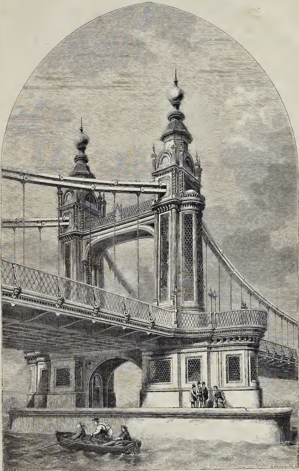
CHELSEA SUSPENSION-BRIDGE.—MR. THOMAS PAGE, ENGINEER.
