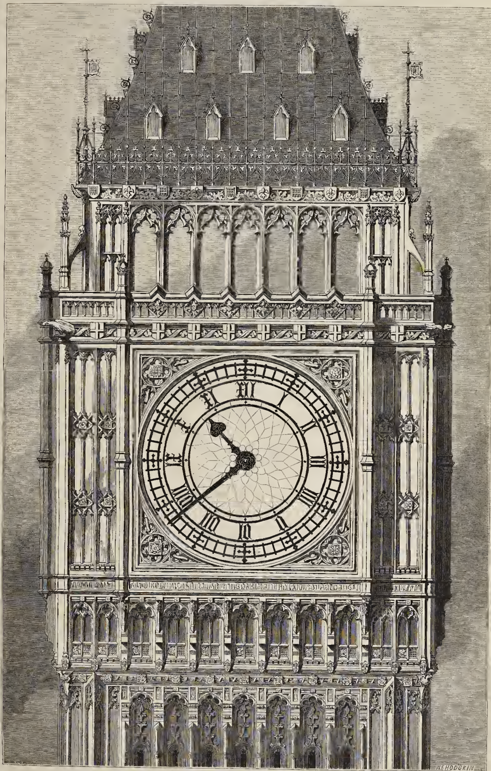
THE CLOCK-TOWER, WESTMINSTER NEW PALACE.—STR CHARLES BARRY, R.A. ARCHITECT.
