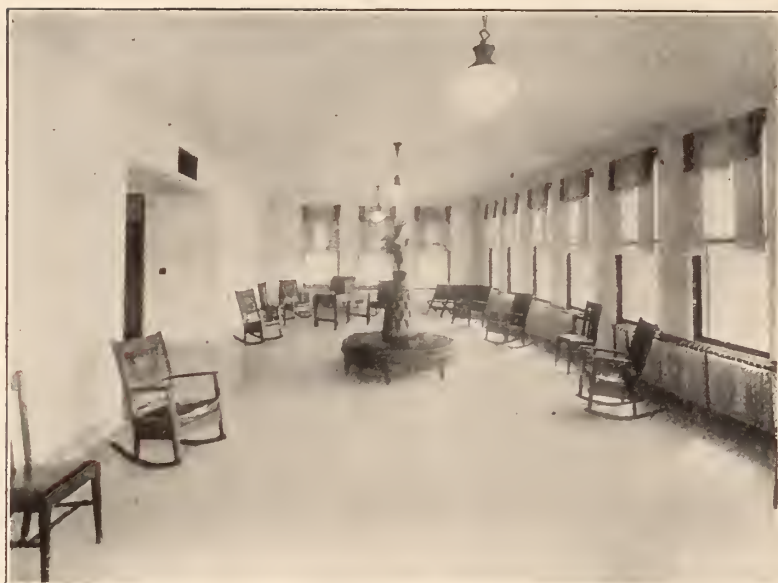
Fig. 3. A "Patients' Day Room," Clark County Asylum. This Asylum, recently completed, cost nearly $1,000,000 and has accommodations for 260 patients. The attractive day room shown in the illustration is certainly in marked contrast to the jail cell with straw and chains of the early days in the state.
