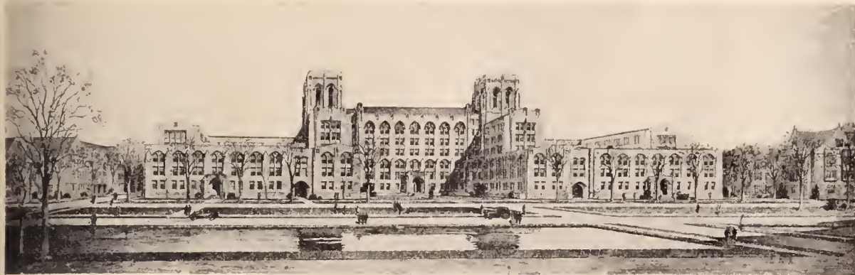
The New Albert Merritt Billings Hospital Under Construction at Rush.
