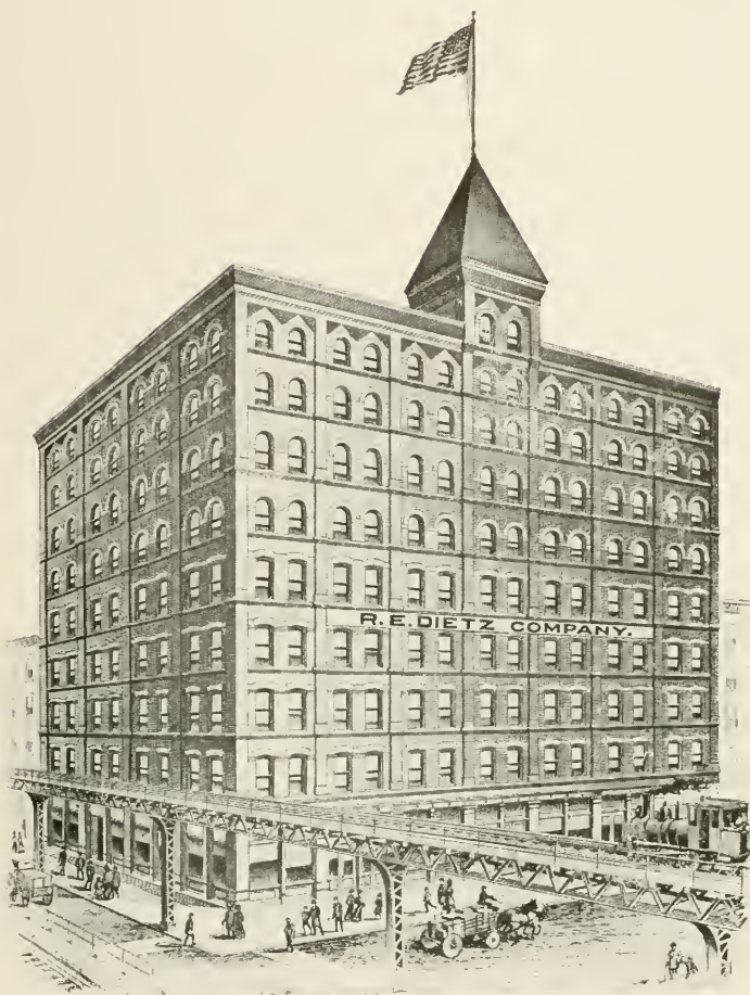
R. E. DIETZ COMPANY'S NEW YORK LANTERN FACTORY, Rebuilt 1898, after the fire; now nine stories, and fire-proof construction Frontage 200 feet. Greenwich at Laight Street, New York City.
