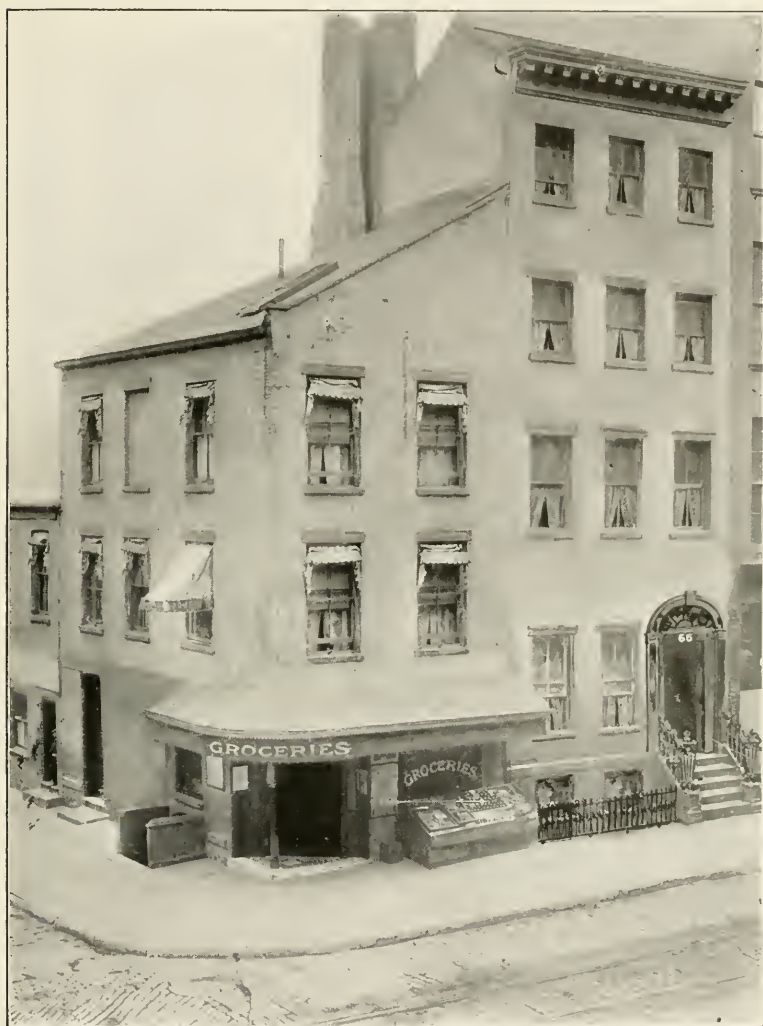
HOUSE No. 66 BEEKMAN STREET
