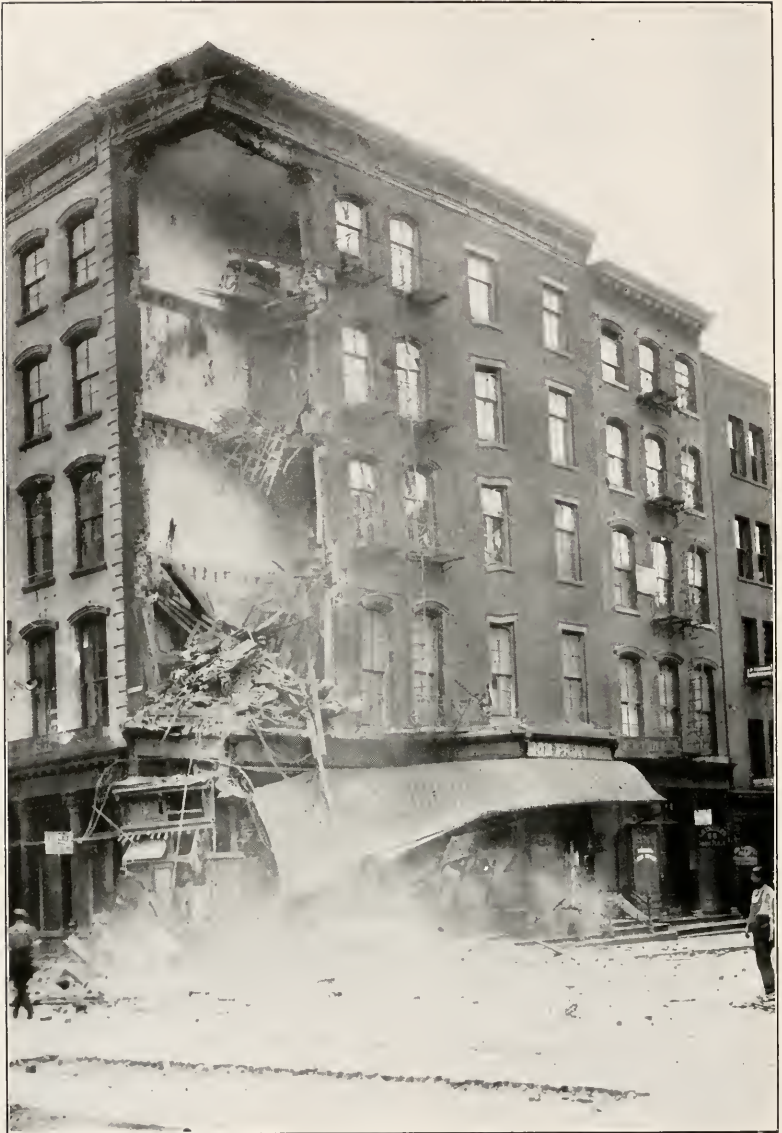
PART OF THE FIRST DIETZ LANTERN FACTORY, After its collapse on June 14, 1910; in it the first Dietz Tubular Lanterns were made.
