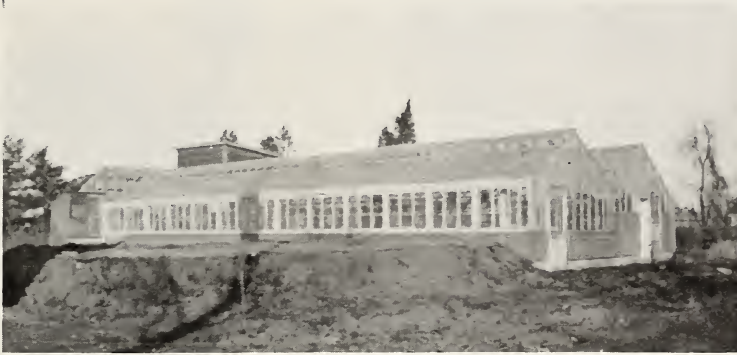
Our Green House Under Construction
