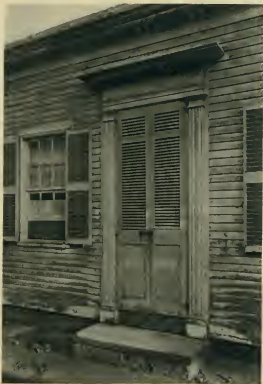
DOORWAY, CORNICE, ETC., OF A LITTLE HOUSE ON ACADEMY HILL, NANTUCKET.
