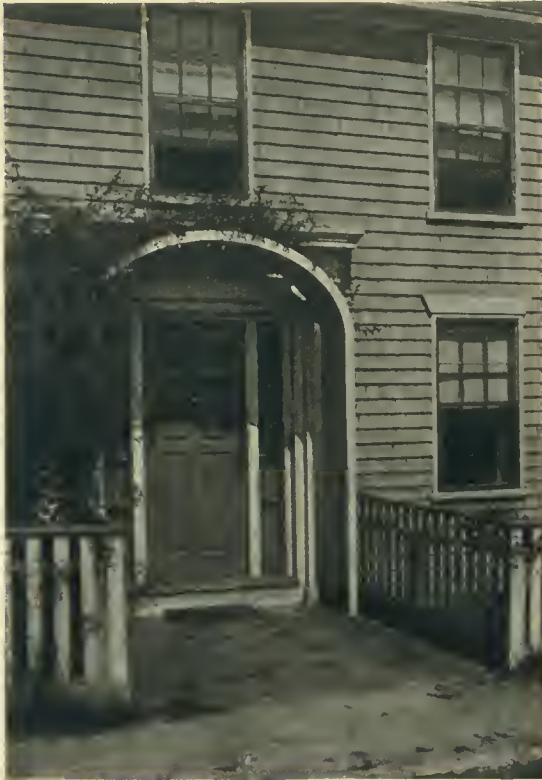
DOORWAY IN QUINCE STREET, NANTUCKET.
