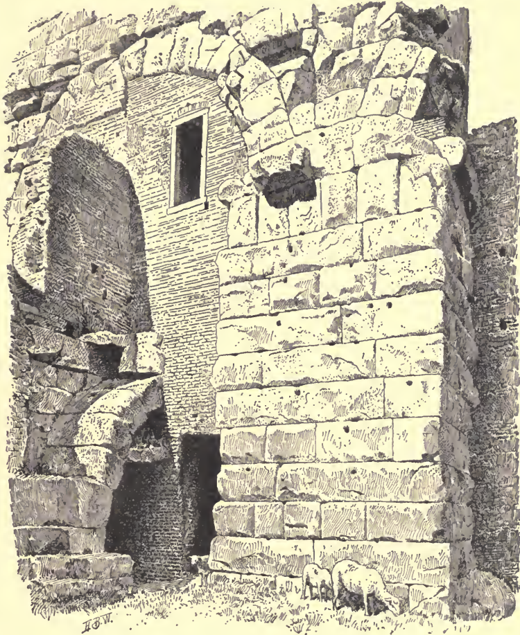
Junction of the Five Great Aqueducts.
