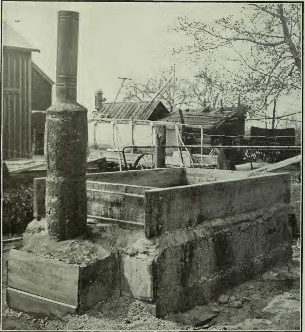
Handy Cooking Plant of 200 Gal. Capacity on Farm of E. Hack, St. Catharines.
