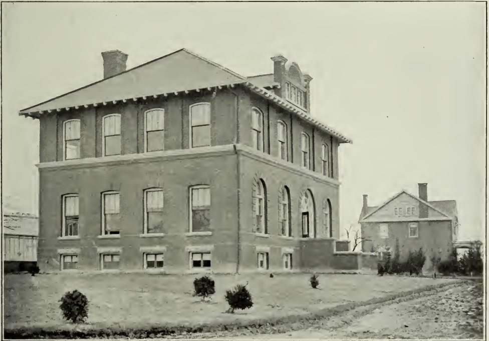
Offices, Laboratories and Directors' Residence at Horticultural Station, Jordan Harbour.
