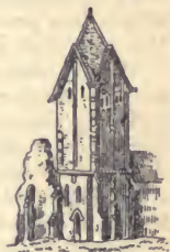
Tower of Sompting Church, Sussex
